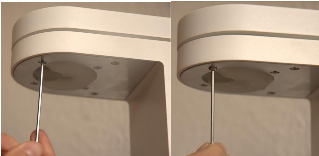
Figure 18: Removal of the Screws From the Bottom Part of the Adapter
